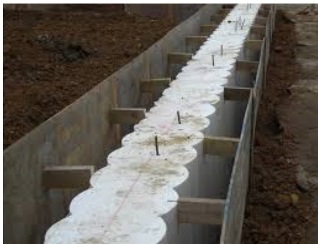
Figure 2: Guide wall ready for concrete
