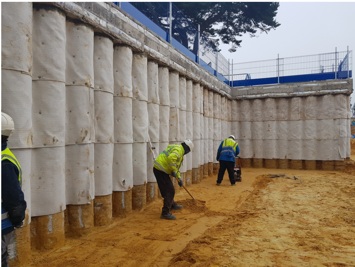
Figure 5: Completed and excavated retaining structure
