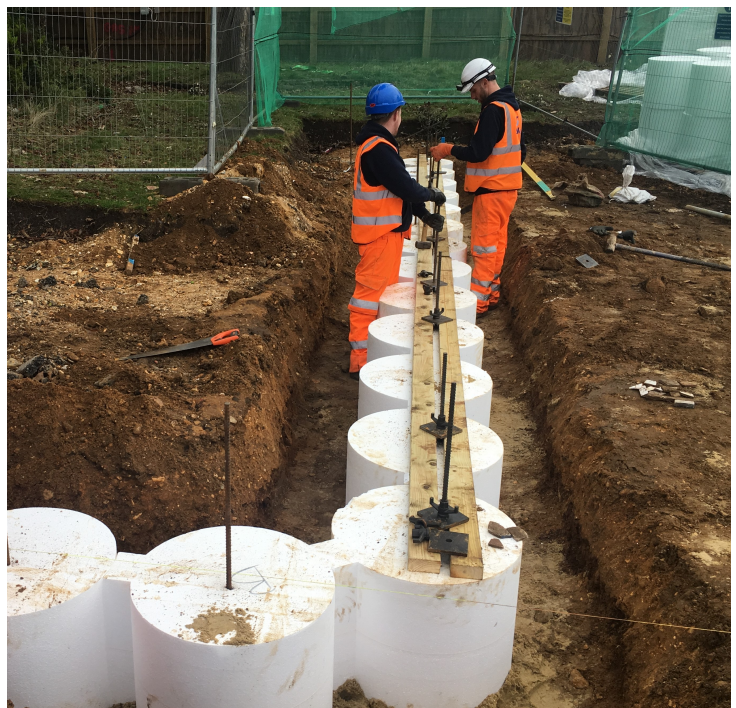
Figure 1: Guide wall formers are placed and tied
