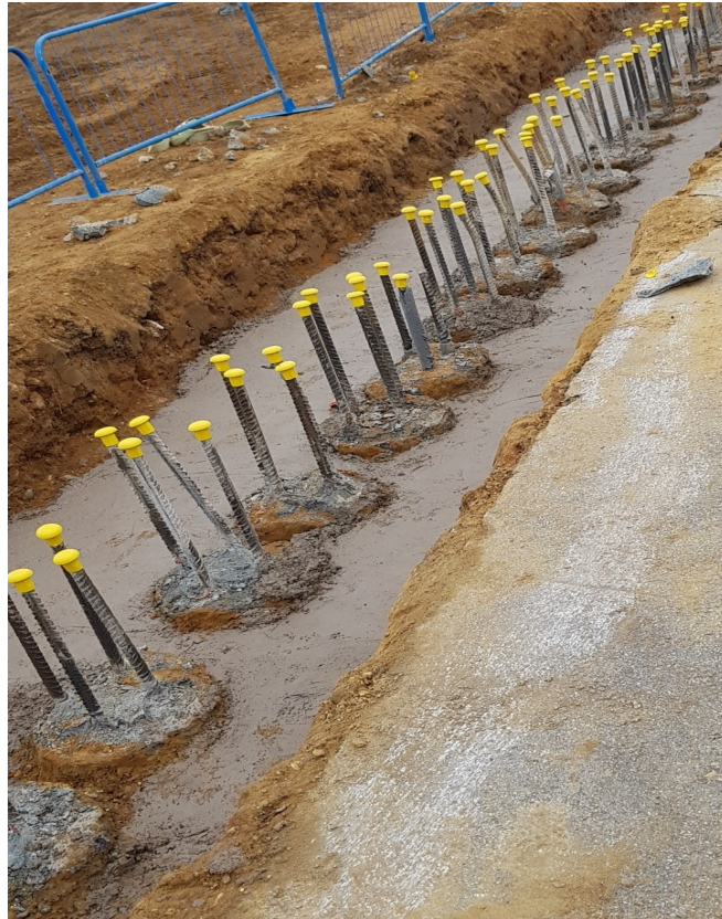
Figure 4: Piles completed and prepared for capping beam
