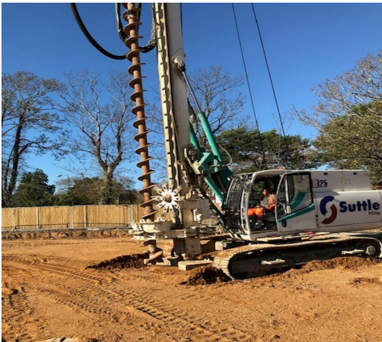
Figure 3: Casagrande B125 piling rig
